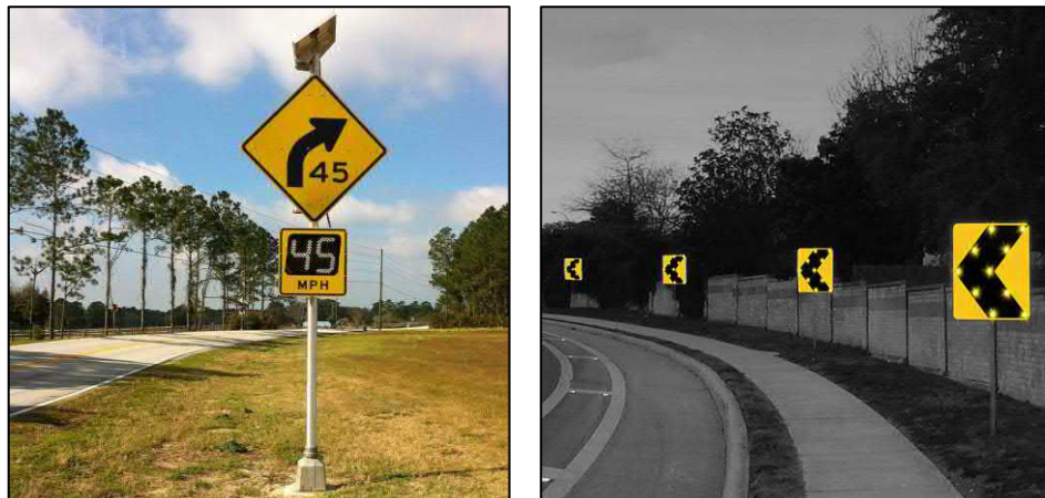
FIGURE 2-3. EXAMPLE DYNAMIC CURVE WARNING SYSTEM SIGNS
