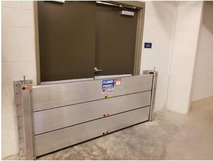
Flood logs as part of a dry floodproofing system
