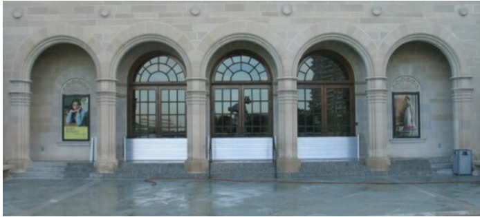
Deployable flood logs at the exterior entrance of a building as part of a dry floodproofing system
