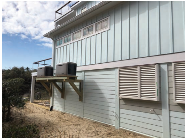
Elevated exterior mechanical systems should be cantilevered off the building when feasible, rather than situated on high platforms extending from the ground.
