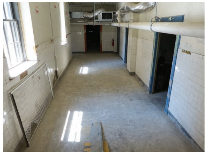
In this building, the mechanical systems in the basement level have been raised above the design flood elevation.
