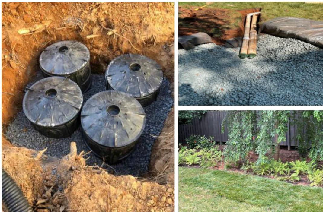
A dry well is a subsurface storage facility that temporarily stores stormwater runoff until it can seep into the surrounding soil. Runoff is stored in a reservoir of gravel, an open-bottomed chamber, or both.
