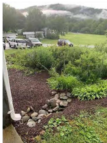
A Rain Garden is a shallow landscaped depression that temporarily ponds stormwater runoff and encourages it to infiltrate into the underlying soil. Rain Gardens are vegetative infiltration practices providing runoff reduction and pollutant removal.
