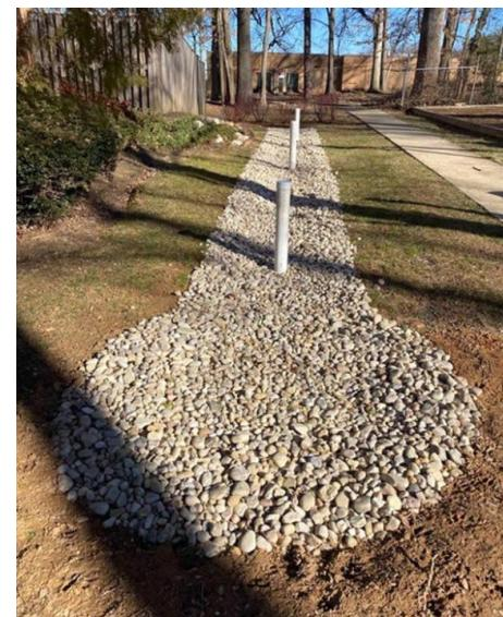
Infiltration practices provide temporary surface and/or subsurface storage of stormwater runoff until it seeps into the ground. Infiltration is a non-vegetative practice that provides runoff reduction. Surface infiltration trenches or basins may utilize a berm to pond runoff; subsurface trenches or basins store runoff in a gravel reservoir, open-bottomed chamber, or perforated chamber. Infiltration does not convey runoff like a French Drain.
