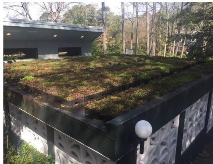
Green Roofs or vegetated roofs are alternative roof surfaces that typically consist of waterproofing and drainage materials and an engineered growth media that is designed to support plant growth. Vegetated roofs capture and temporarily store stormwater runoff in the growth media. A portion of the captured stormwater evaporates or is taken up by plants, which helps reduce runoff volumes, peak runoff rates, and pollutant loads on development sites.
