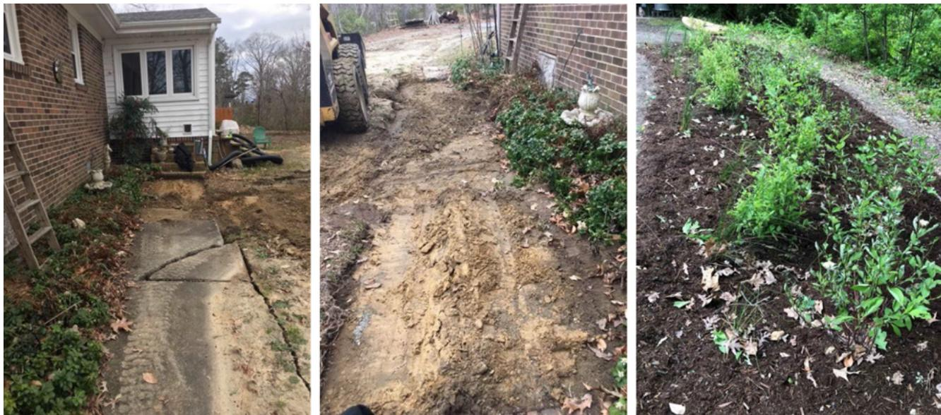
Impervious Surface Removal is the demolition and disposal of impervious surfaces and includes remediation of the subsoil, adding topsoil, and vegetation establishment or other best management practice. Impervious surfaces include hardscape and pavement materials such as asphalt, concrete, brick, and densely graded stone aggregate.
