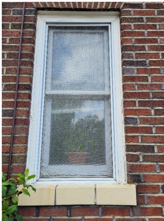
Window A – Brick moulding has minor water damage on both sides.
