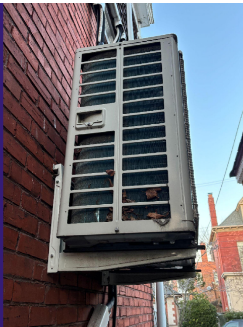
Photograph of mini-split and mounting brackets.
