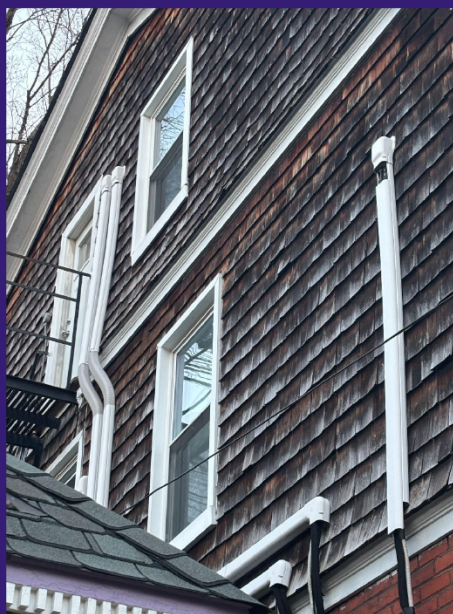
Photograph of conduit lines.
