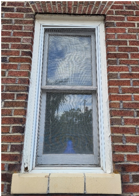
Window B –Brick moulding has damage at bottom left side.
