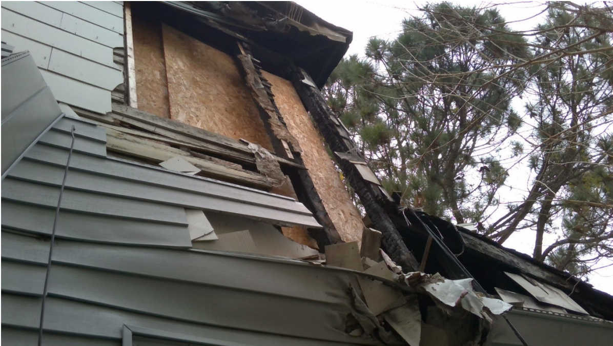
Damaged east elevation and rear addition showing asbestos and wood siding beneath vinyl siding, 11/20/2025.
