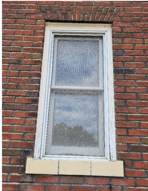
Window H –Brick molding has damage on both sides at bottom.
