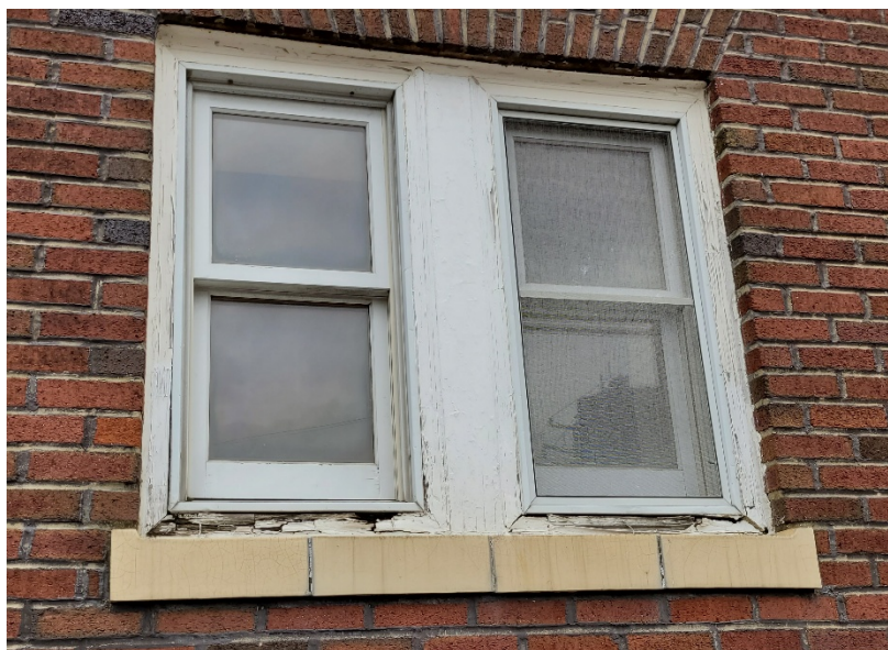
Window G –Brick moulding is extensively deteriorated underneath both windows.
