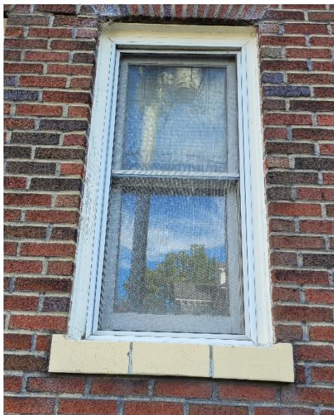
Window M –Brick moulding has minor deterioration at bottom left side.
