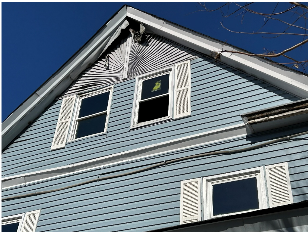
Fire damage in upper front gable, 1/29/2026.
