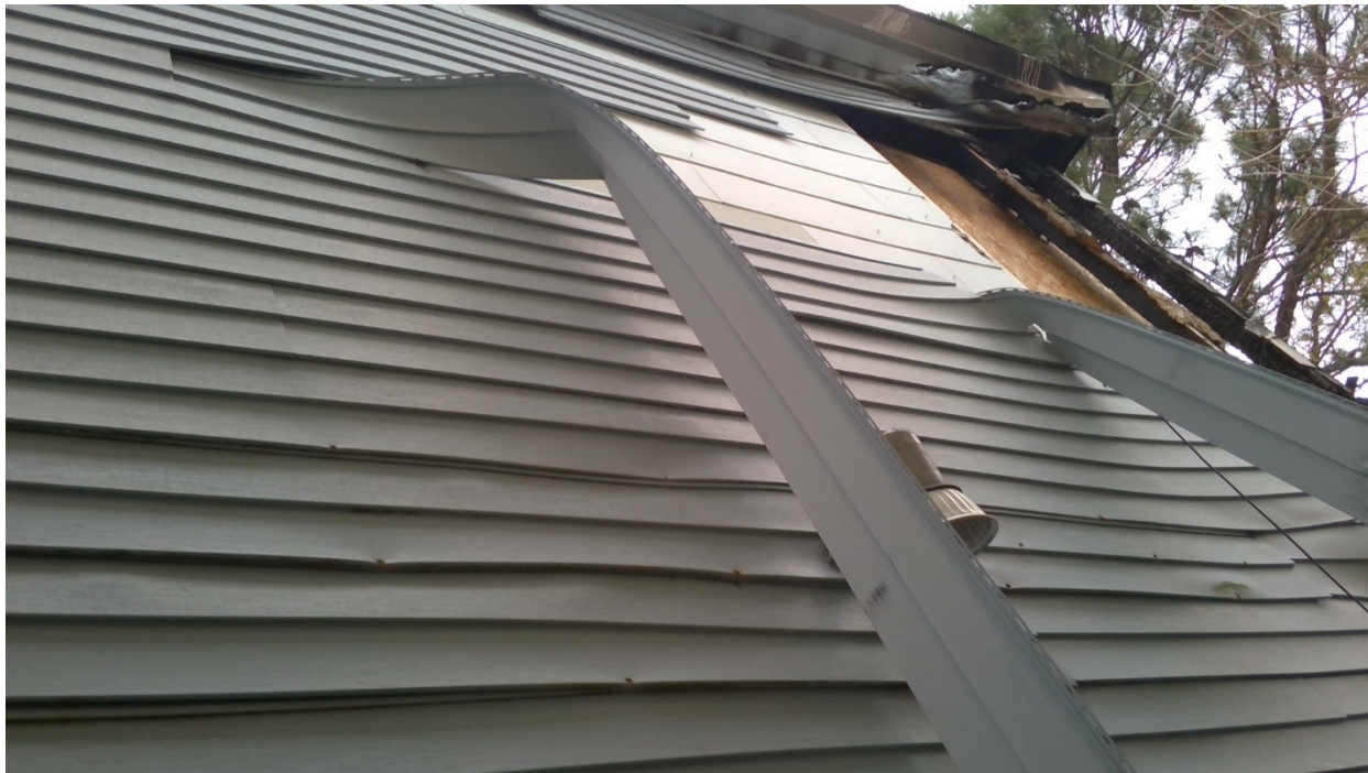
Damaged east elevation and rear addition showing asbestos siding beneath vinyl siding, 11/20/2025.
