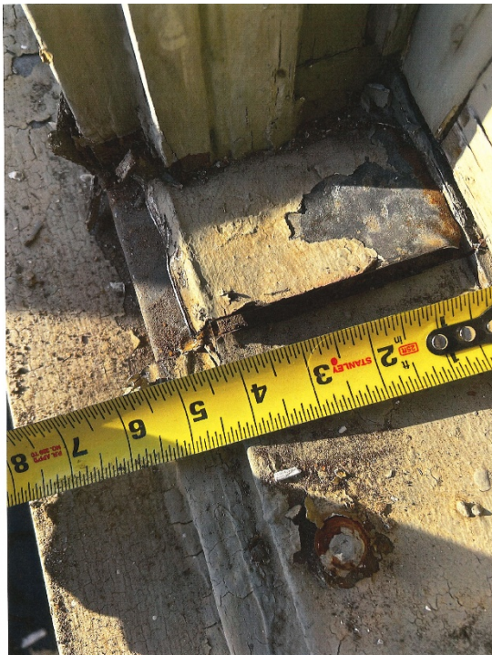
Existing window sill with metal wrap.
