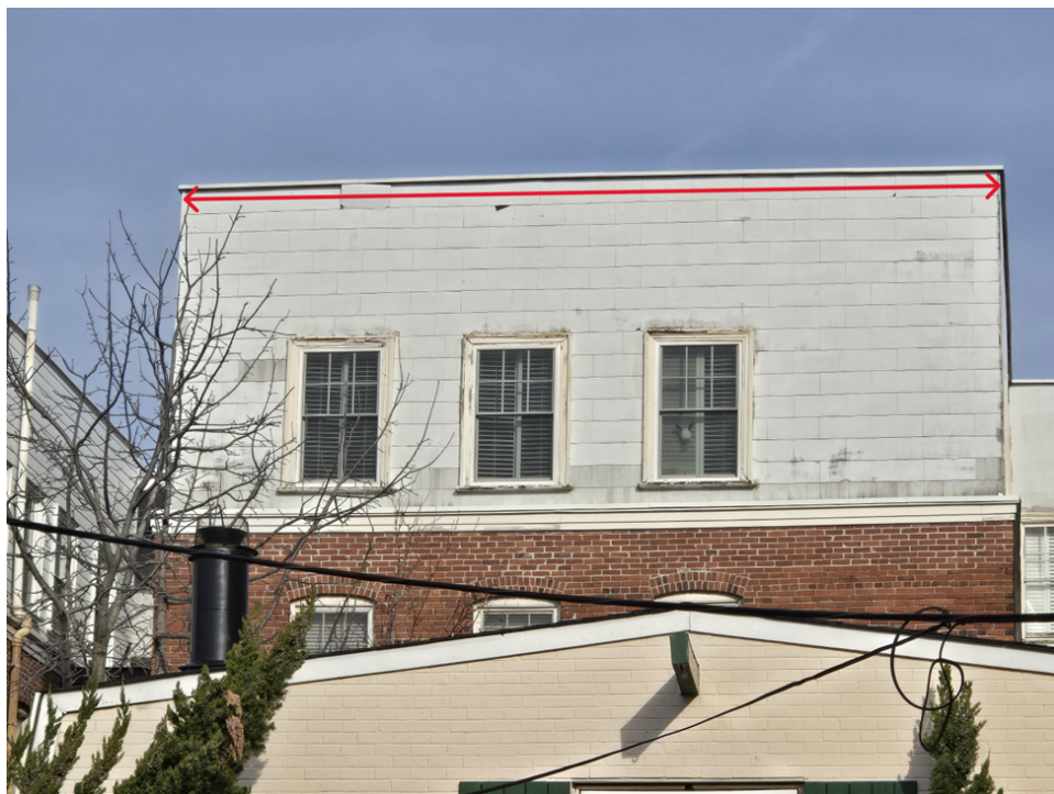
Rear elevation with asbestos siding that will be replaced, December 2025.
