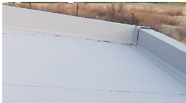
TPO ROOFING MEDIUM-DARK GREY, THERMOPLASTIC POLYOLEFIN
